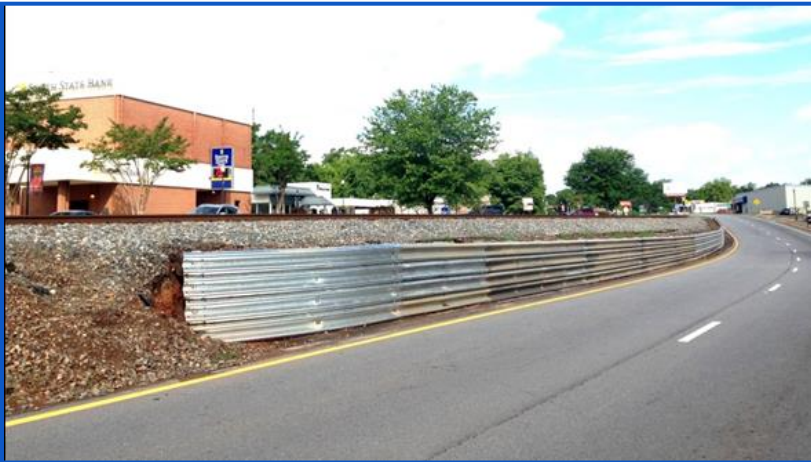
Retaining wall repair on Broad St.
