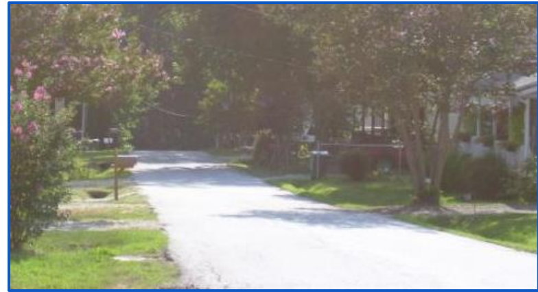
A traditional neighborhood without sufficient pedestrian amenities.
